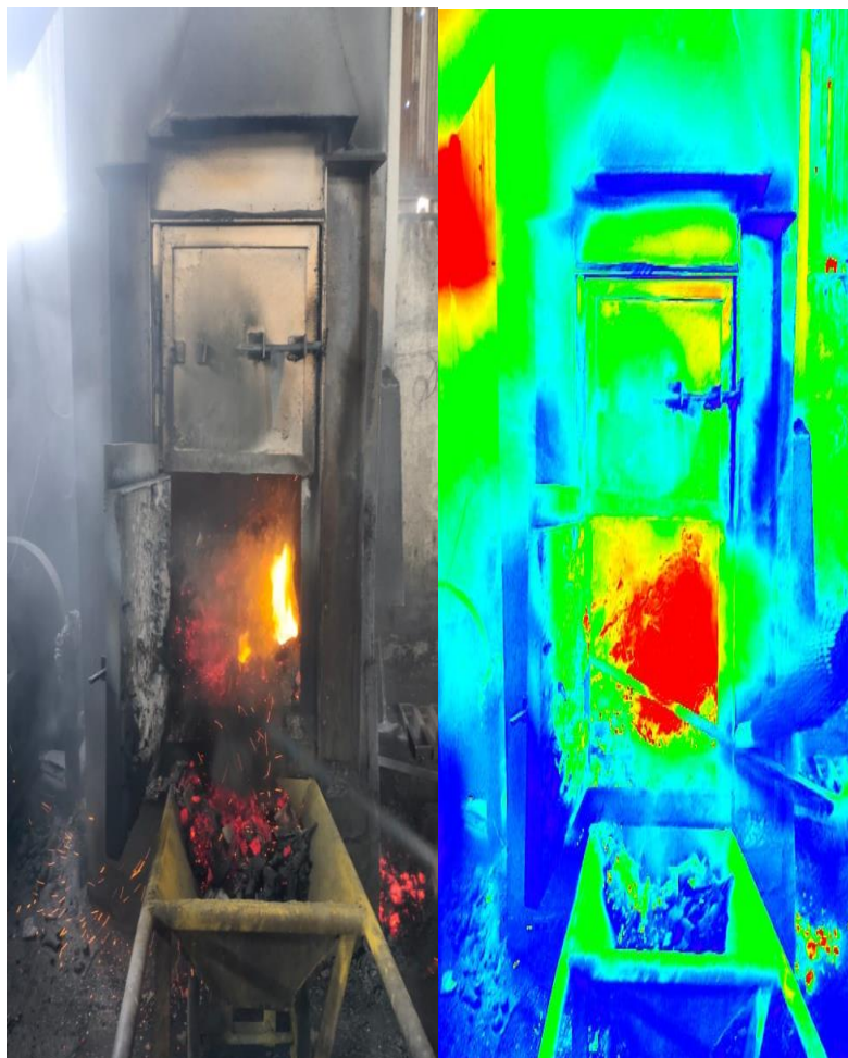
Fig.5.1 and Fig.5.2 CUPOLA FURNACE'S THERMAL IMAGES.
